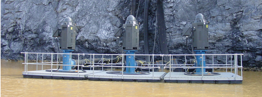
3 pumps on 3 floating platforms attached together.
