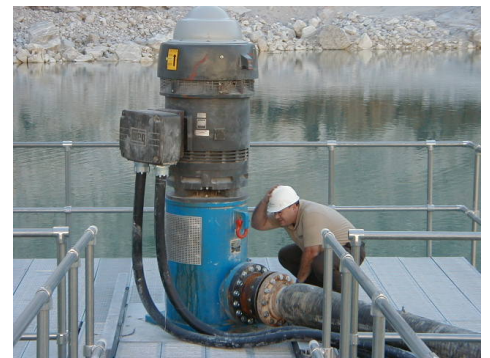
Large vertical pump with walkway.
