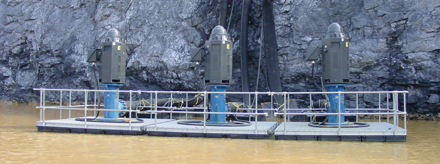
3 pumps on 3 floating platforms attached together.
