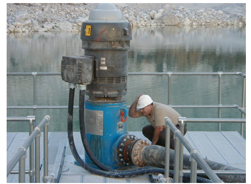
Large vertical pump with walkway.
