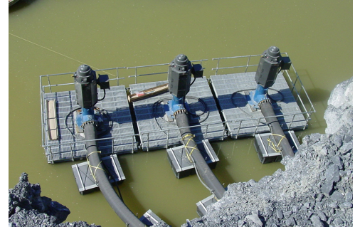
Large vertical pump with walkway.
