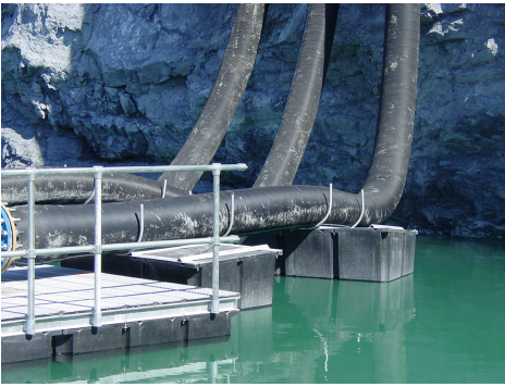
Pipe line float carrying 18" pipe from pump
