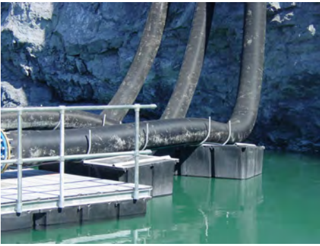
Pipe line float carrying 18" pipe from pump
