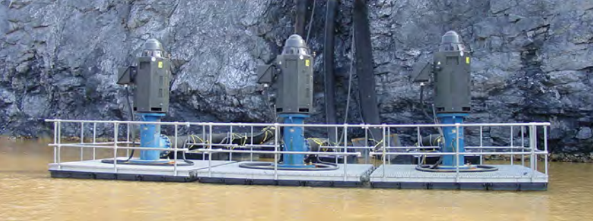
3 pumps on 3 floating platforms attached together.
